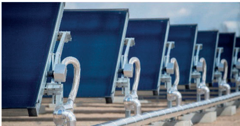
Flat Plate Collectors (© Newheat)
